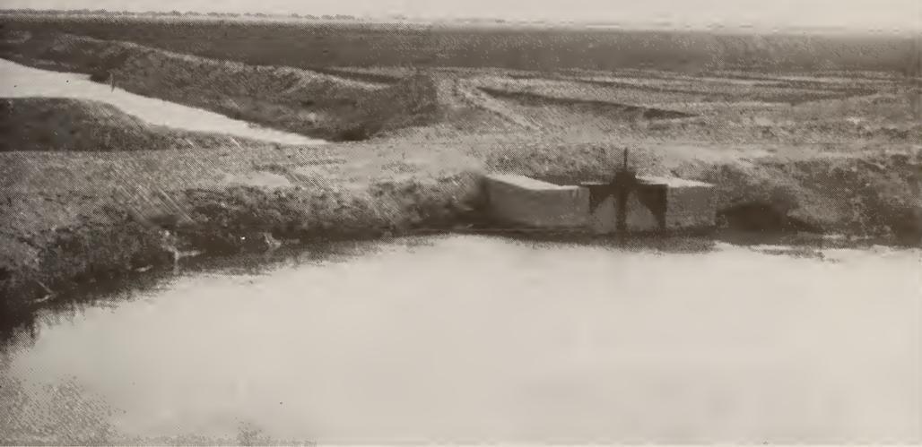
*Control device for switching water flow to one of the many canals used for irrigation in Al Jazirah, south of Khartoum
